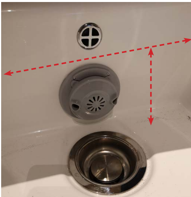
A. The water level must ALWAYS COVER THE HYDROMASSAGE MAGNA JET
