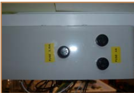
Fig. 1 – Fuse for Cromo (3.15A or 4A) and electronic card (4A or 6,3A)
